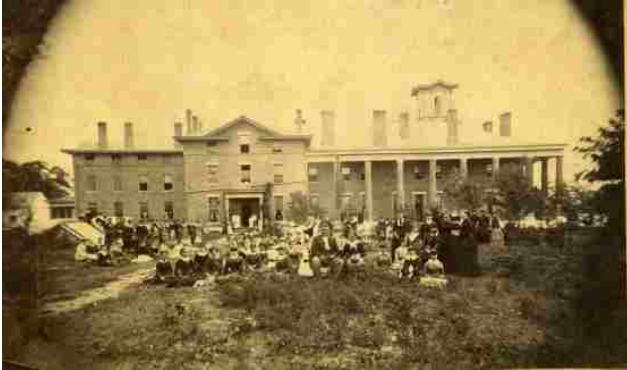
Figure 31: Cherokee Male Seminary, Tahlequah, Oklahoma, 1846-51, with 1875 addition on left. Courtesy of Oklahoma Historical Society, ca. 1875-1908.
